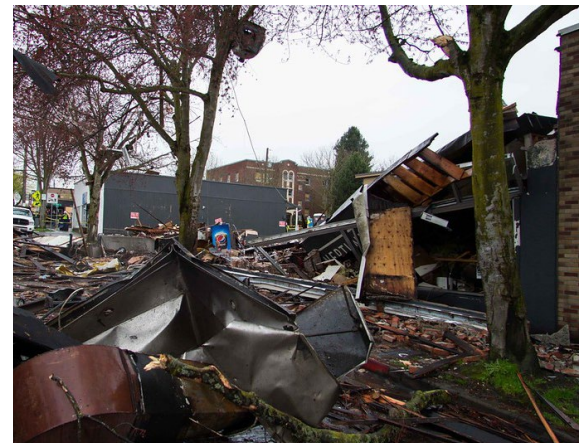
Greenwood pipeline explosion in 2016
