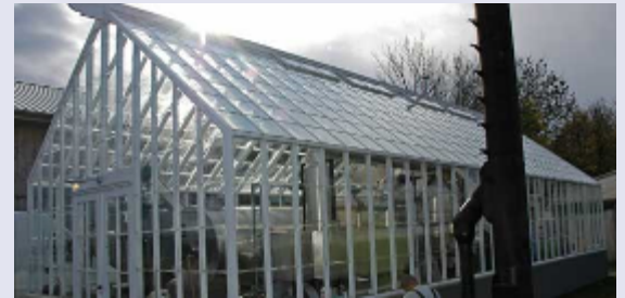
Greenhouse, boiler, biochar stirling engine (DK)
