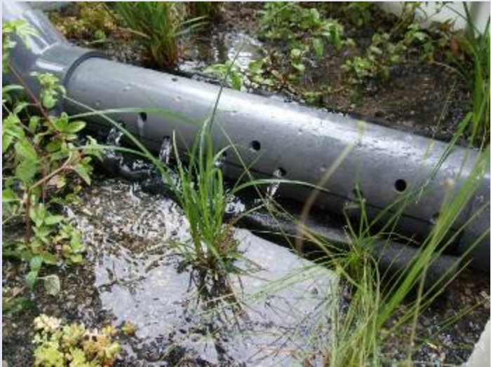
Improved storm water quality
