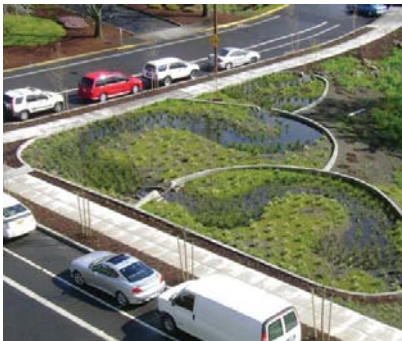
This rain garden in Portland, OR treats storm water from adjacent development and right-of-way, filtering pollutants as well as slowing and reducing volume of stormwater flows.
