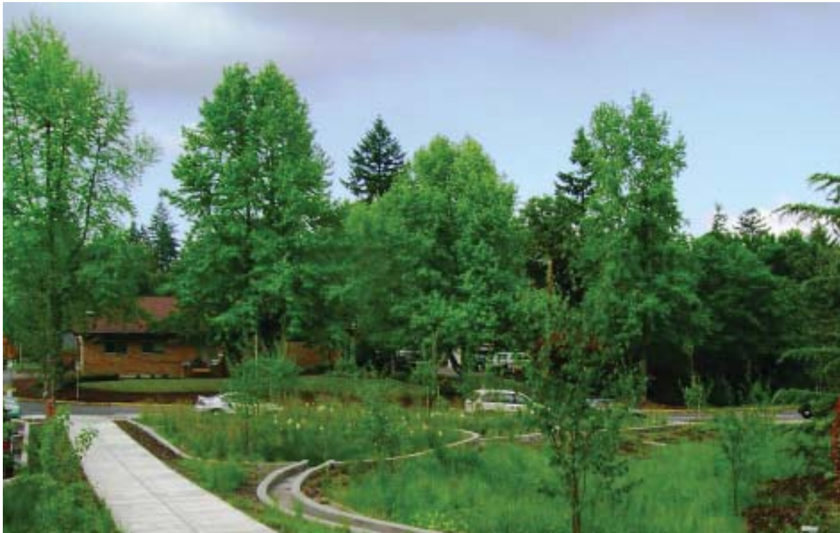
A rain garden in Portland, Oregon treats storm water from adjacent development and right-of-way, helping to filter pollutants as well as slowing and reducing the volume of stormwater flows
