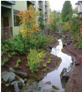
A daylighted stream in Portland, OR connects an upstream forested wetland with a downstream rain garden and directs flow below the surface for groundwater recharge.
